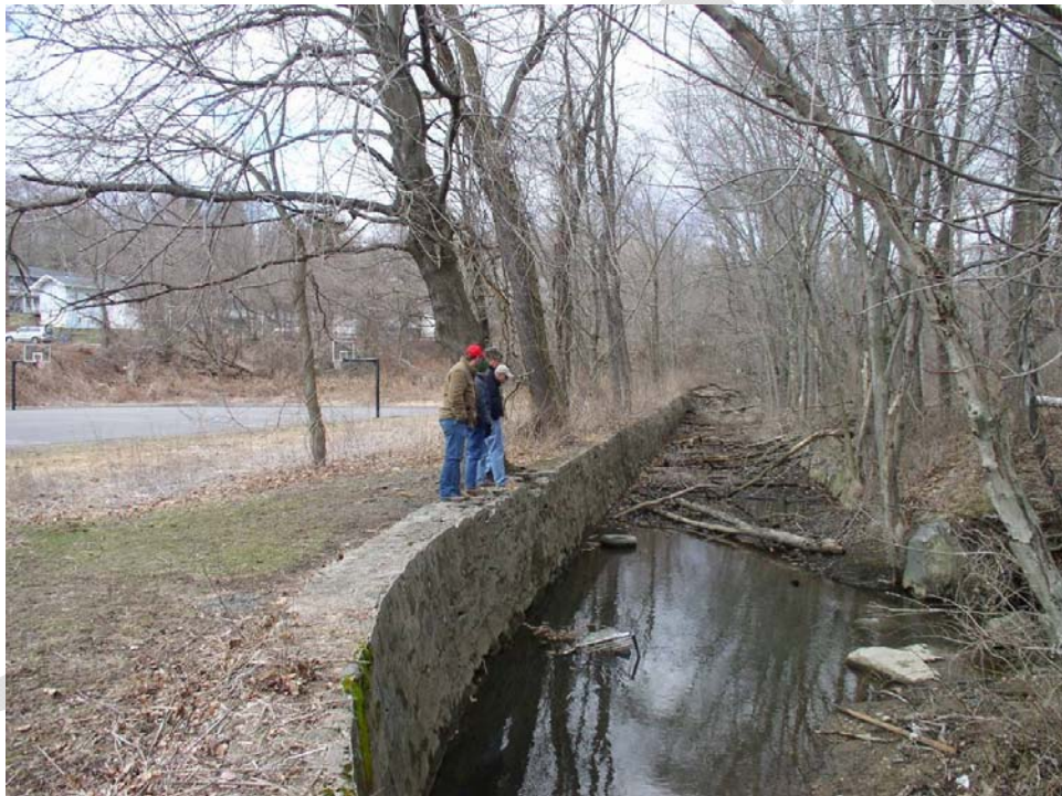
Figure 12: Historic rock channel and side wall. (Photo courtesy of Carol Donzella, NRCS Community Planner)
